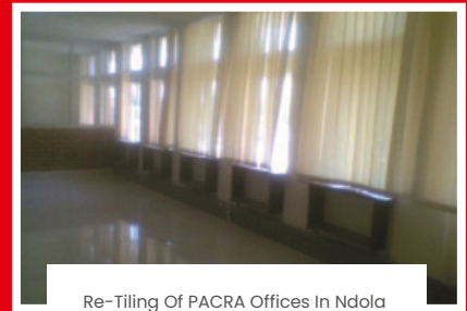
Re-Tiling Of PACRA Offices In Ndola
